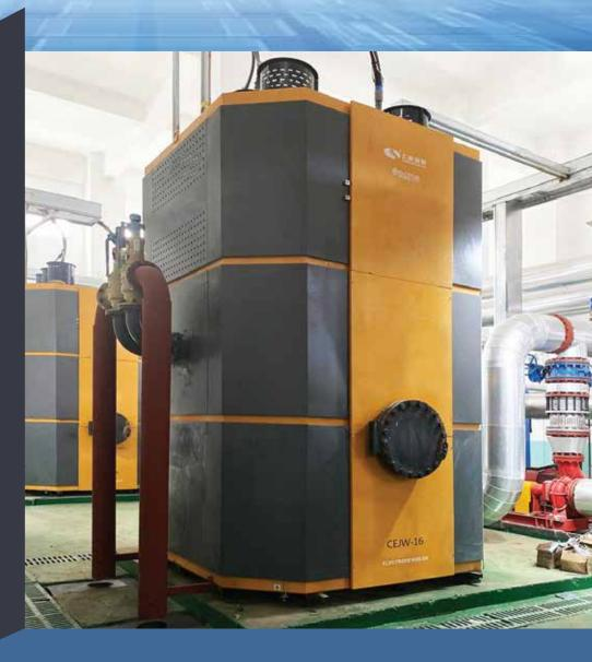
HIGH VOLTAGE IMMERSED ELECTRODE HOT WATER BOILERS
