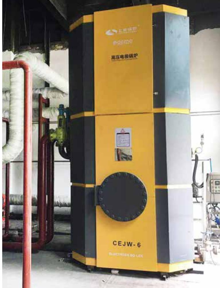
equipment, saving on capital expenditures. Also, in the case of using Electric Boiler, they eliminate the need for a stepdown transformer.
